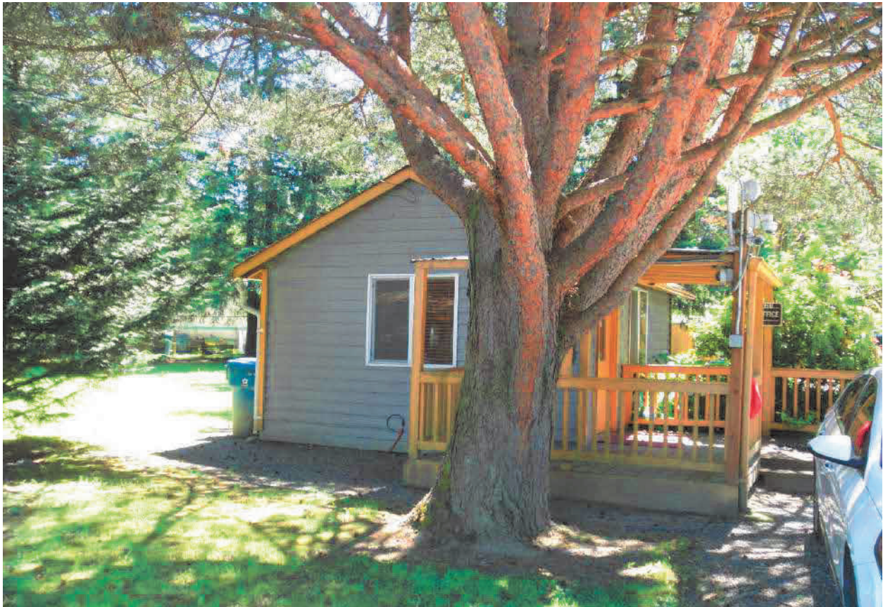
View of the Office
