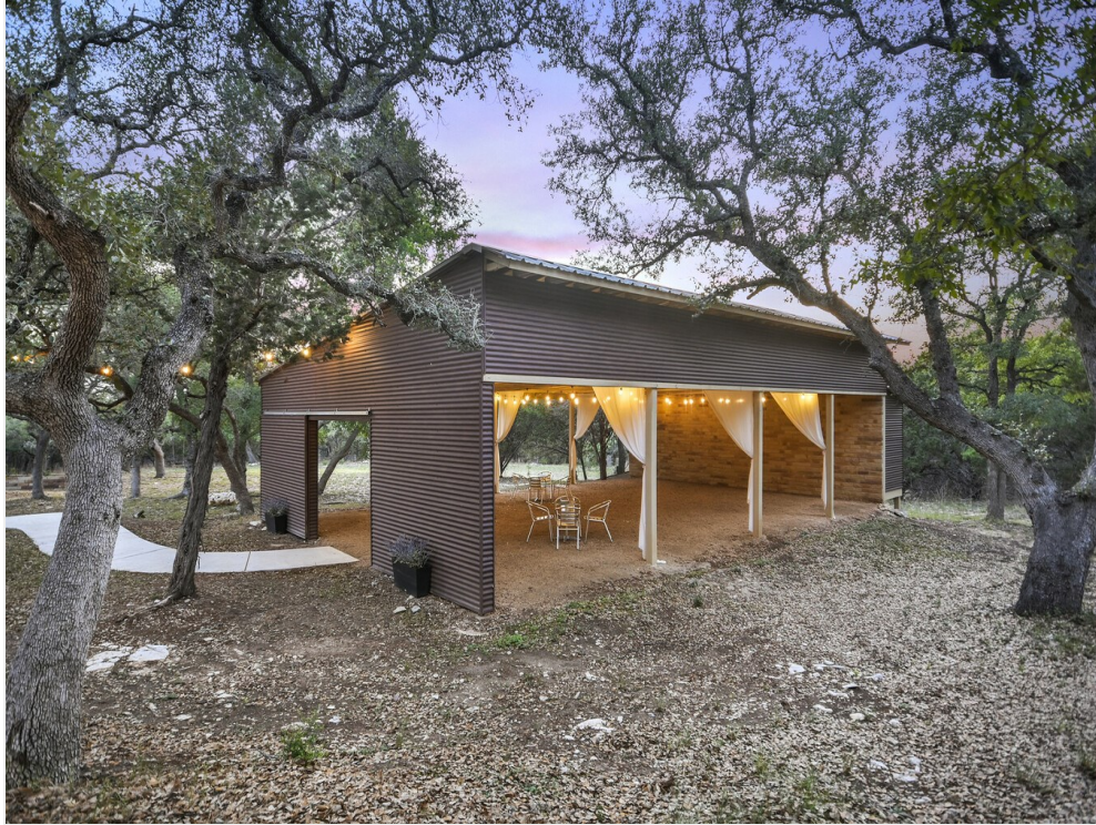
Open Air Pavilion
