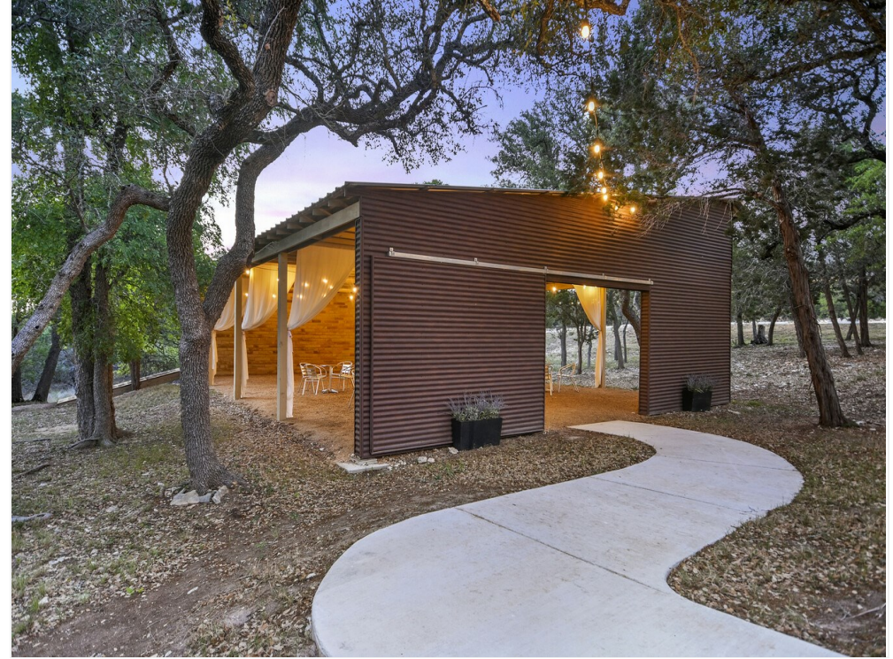
Open Air Pavilion
