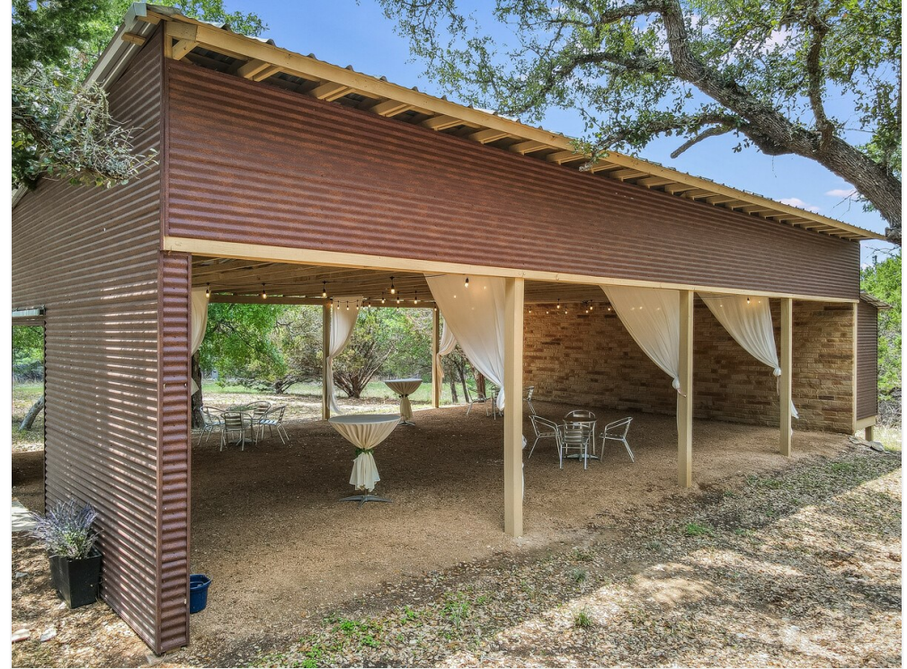
Open Air Pavilion
