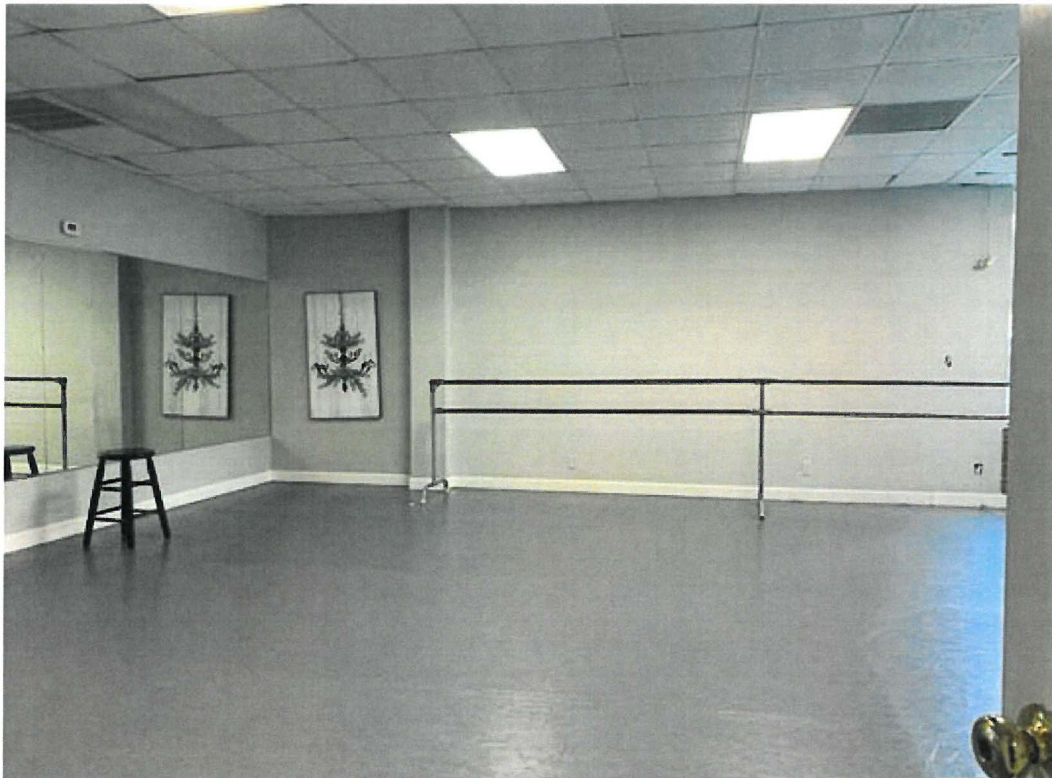
VIEW OF LARGE ROOM
