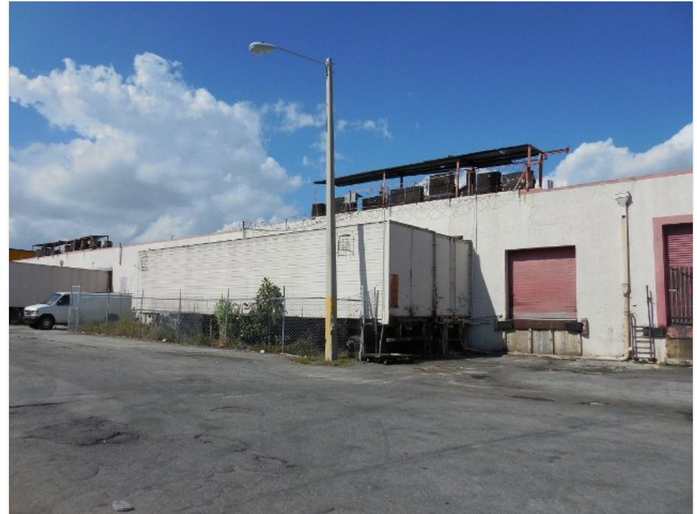
View along NW 22 Terr
