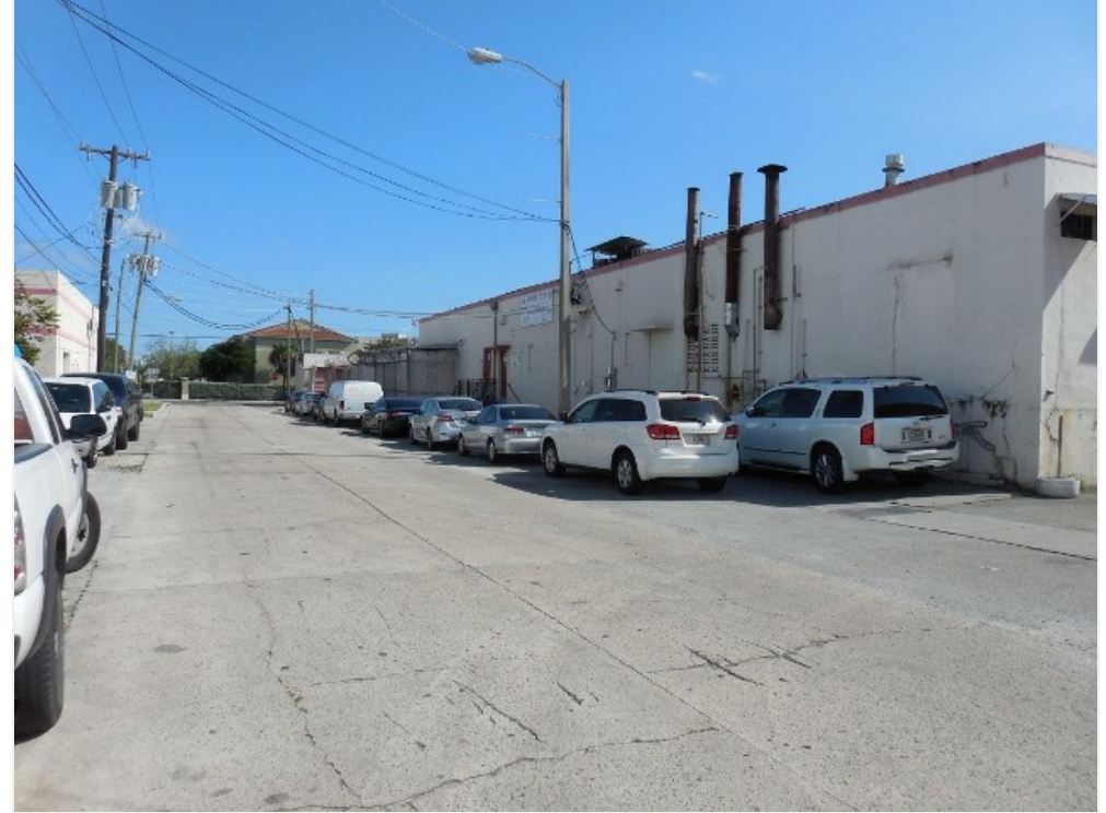
Meat Processing Plant Building (3)
