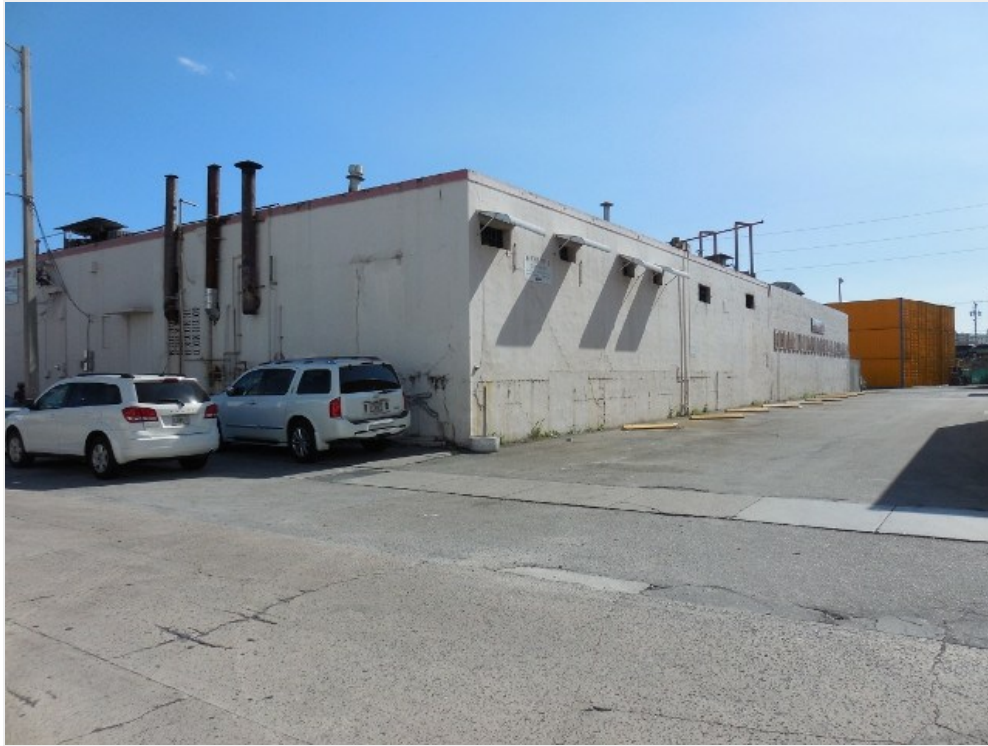
View from the West on NW 23 St
