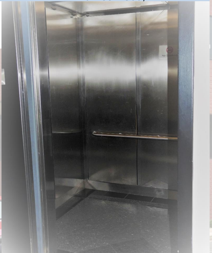
Renovated Elevator Cab
