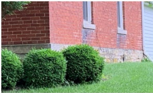
Example of original stone foundation
