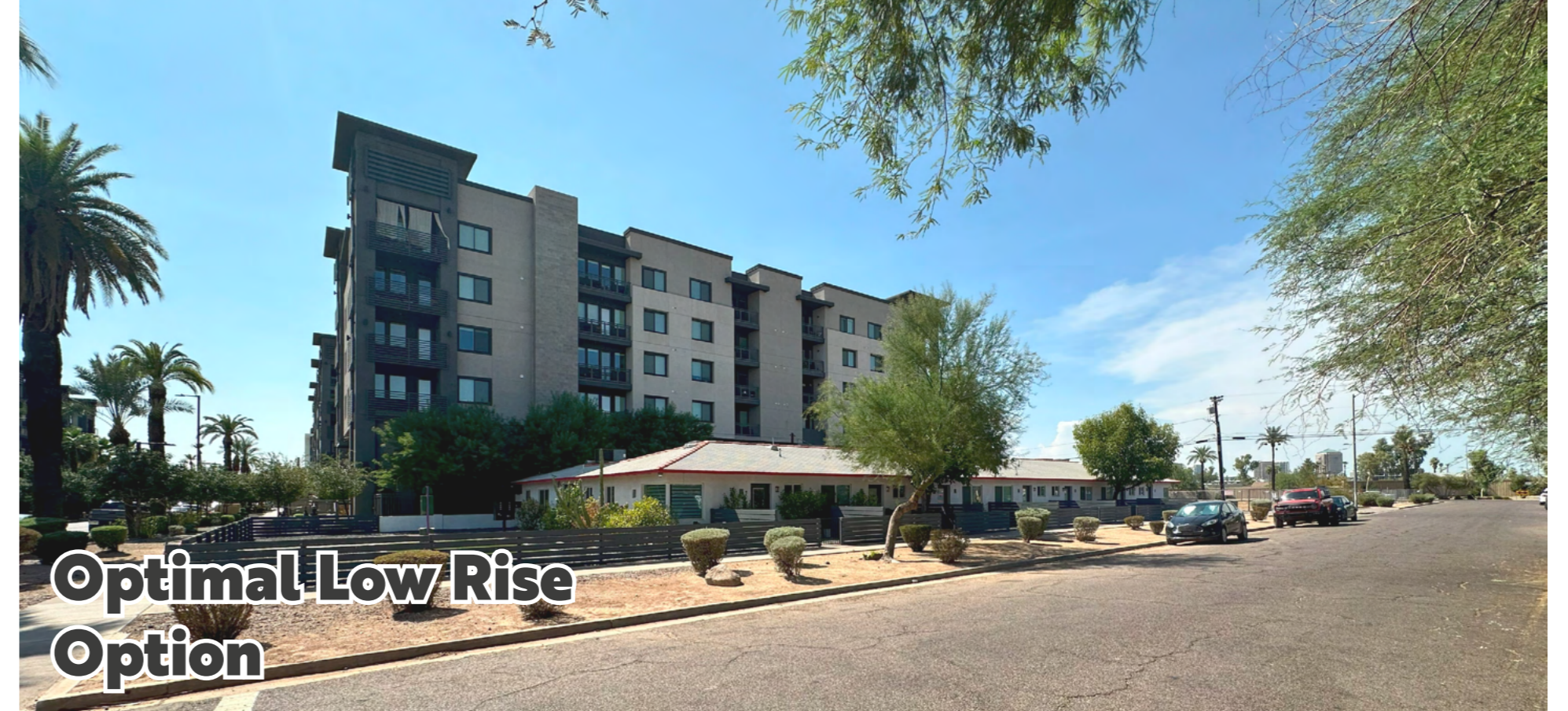
Low Rise Redevelopment Option up to 5 floors in height may reduce the building cost for optimal ROI but with smaller income streams compared to the high and mid rise options. Please see the feasibility projection analysis table (pg. 12-13) on how 465% ROI may be possible with this option.
