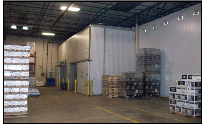
Skewed View Of The "Cool" Room
