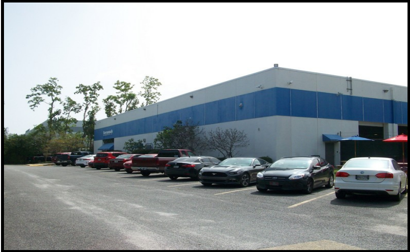
Easterly View Along The Northern (Front) Elevation
