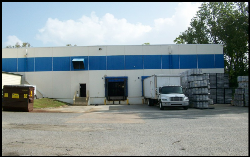
View Of A Southerly Portion Of The Western Elevation
