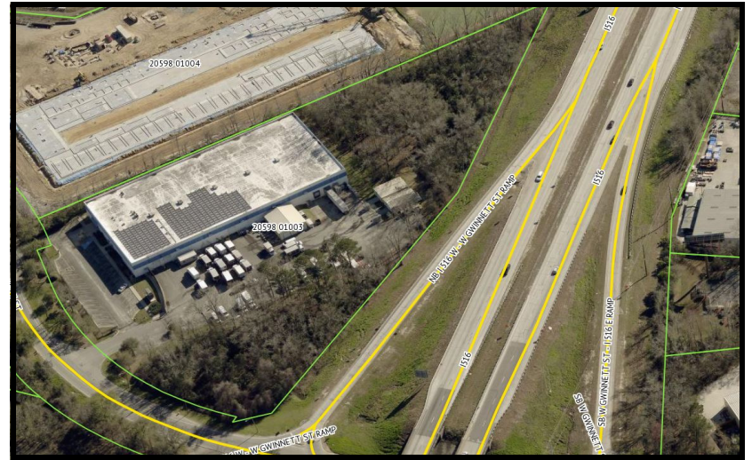
SOUTHEASTERLY AERIAL VIEW
