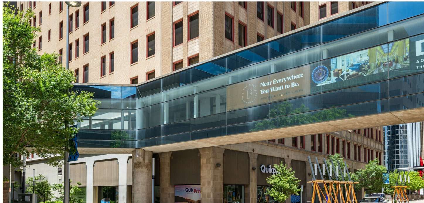
Skybridge Connecting to the SE Side of Building
