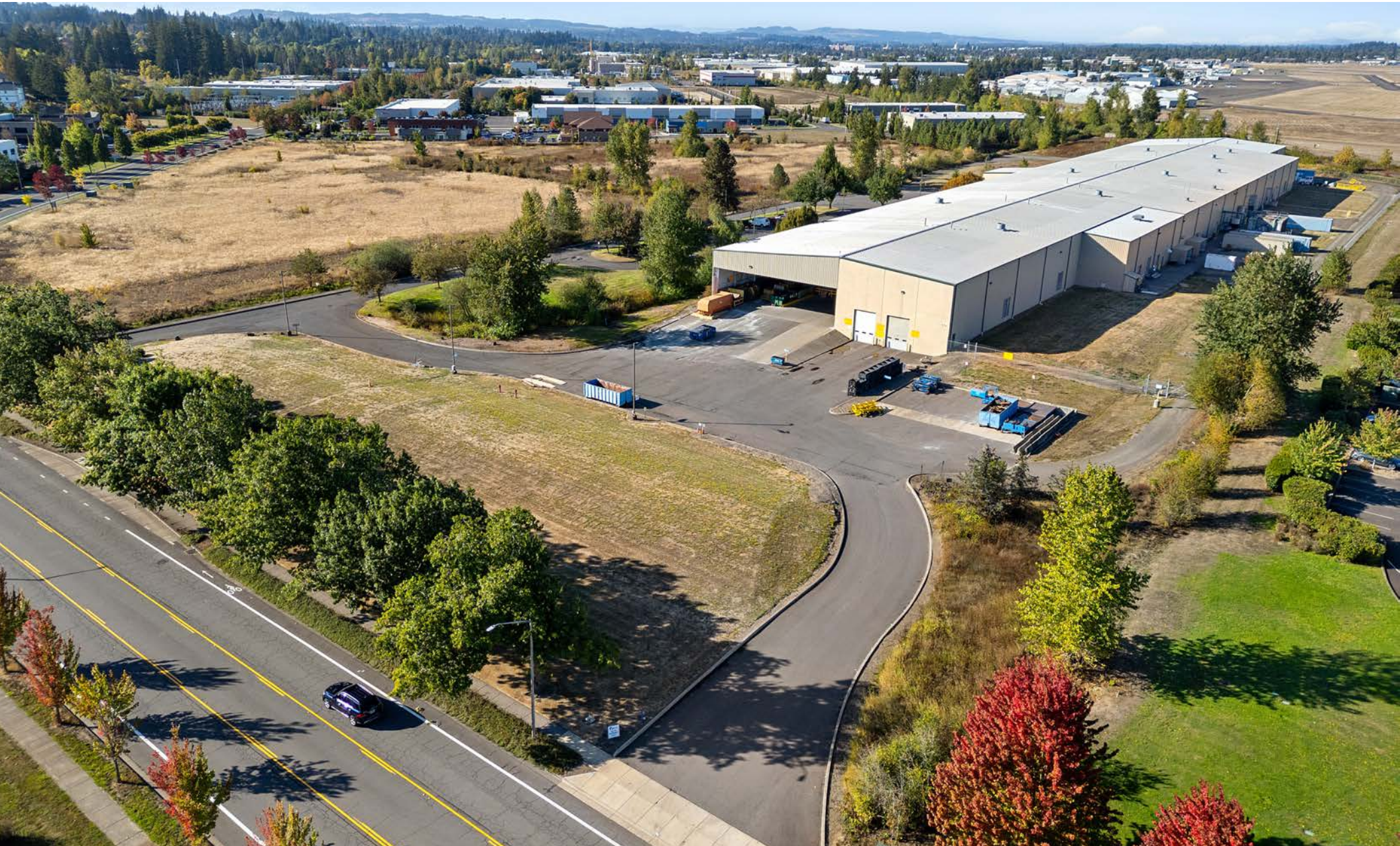
VITRO SALEM INDUSTRIAL BUILDING
