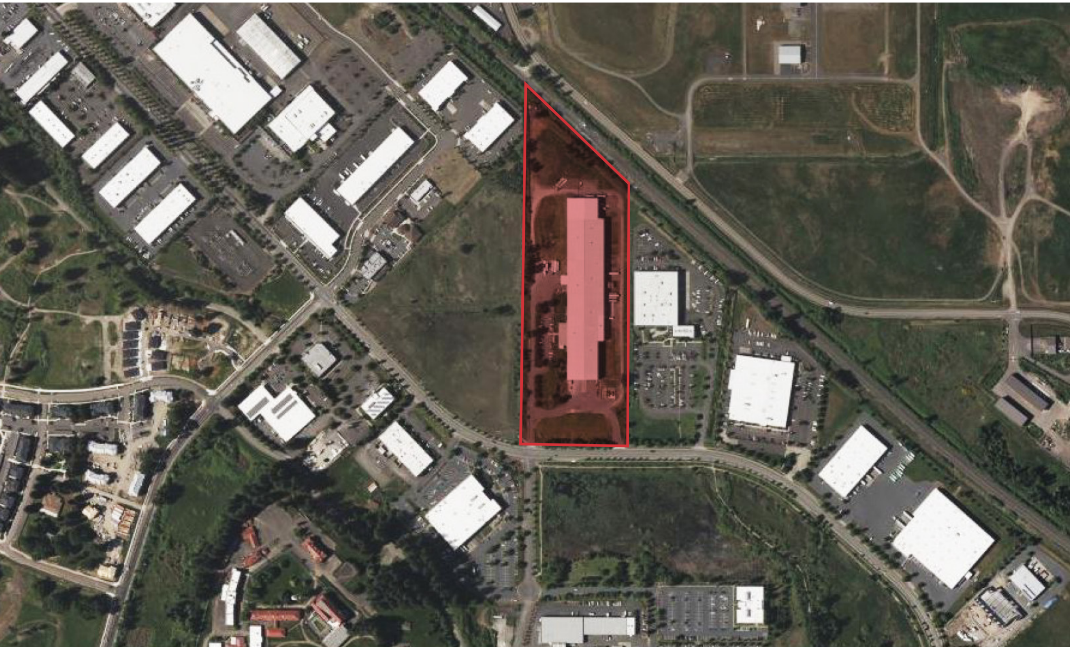
VITRO SALEM INDUSTRIAL BUILDING
