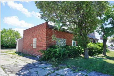
E. side view of the brick building.
