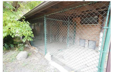
View of detached kennel area
