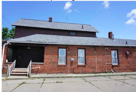
W. side of the brick building.
