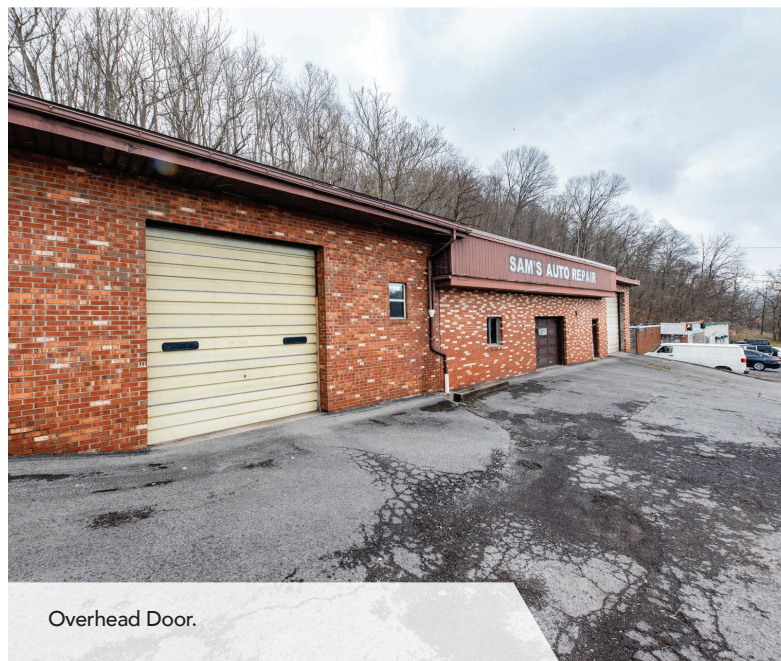
Front of Industrial Building.
