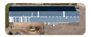
This industrial commercial building was built in Steel, on 16' concrete slab with 10' x 10' deep concrete sections at each steel beam.
