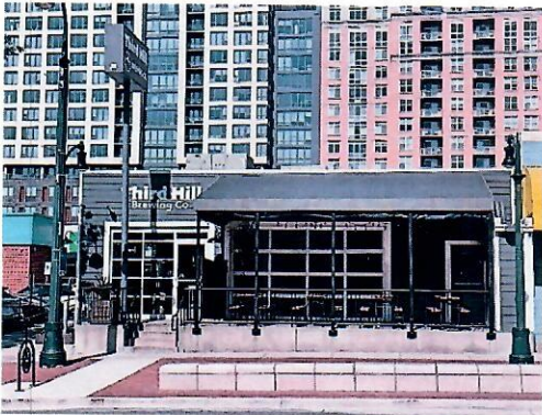
8216 Georgia Ave. Front view from Georgia Ave.
