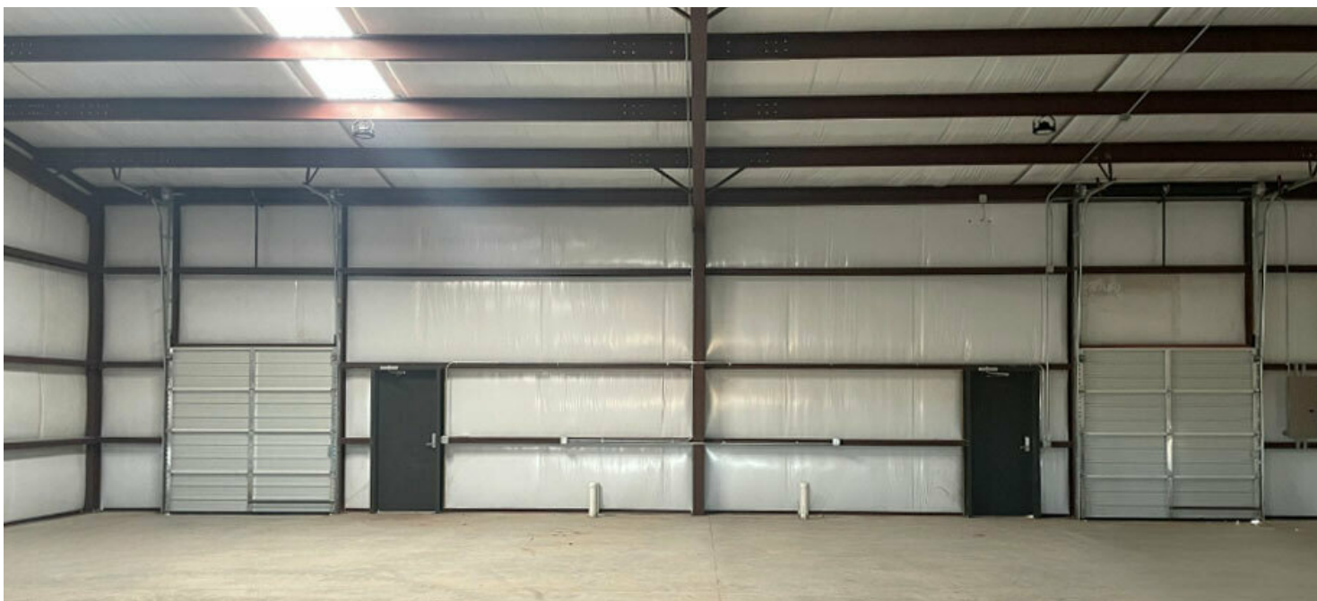
Rear Overhead Doors
