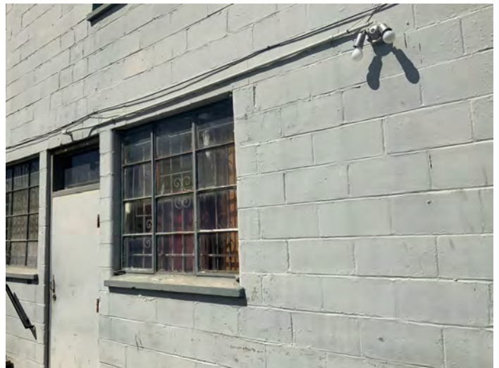
Rear of Structure
