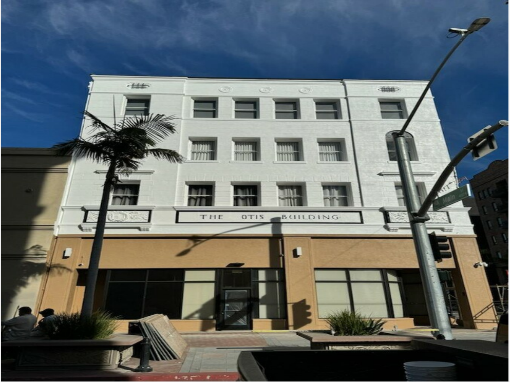
Exterior 4th St.
