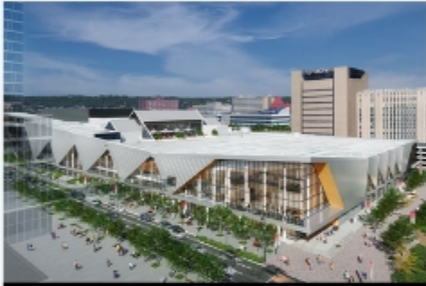
Convention Center Renovation Full Office Renovation
