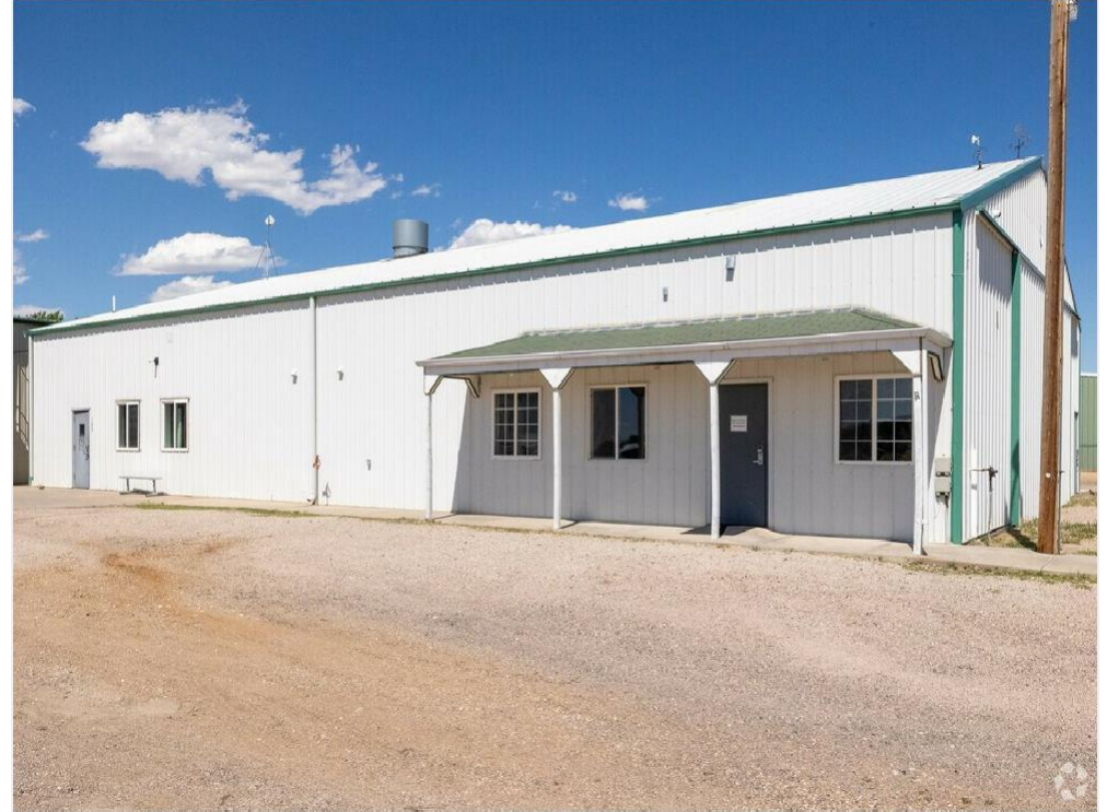
SECONDARY WAREHOUSE WITH PAINT BOOTH
