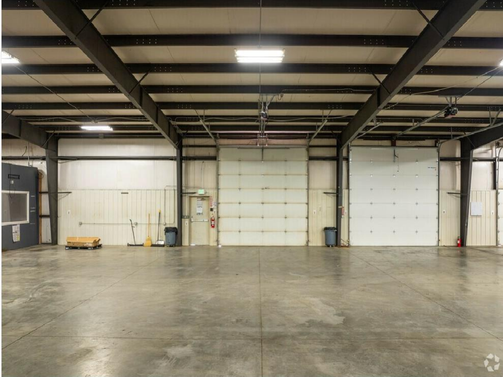
MAIN WAREHOUSE-OVERHEAD DOORS-X4
