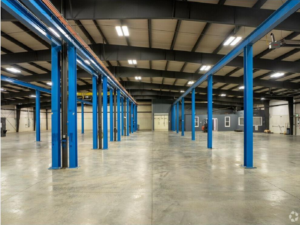
MAIN WAREHOUSE-CRANES/OVERHEAD DOOR ACCESS TO MACHINE SHOP
