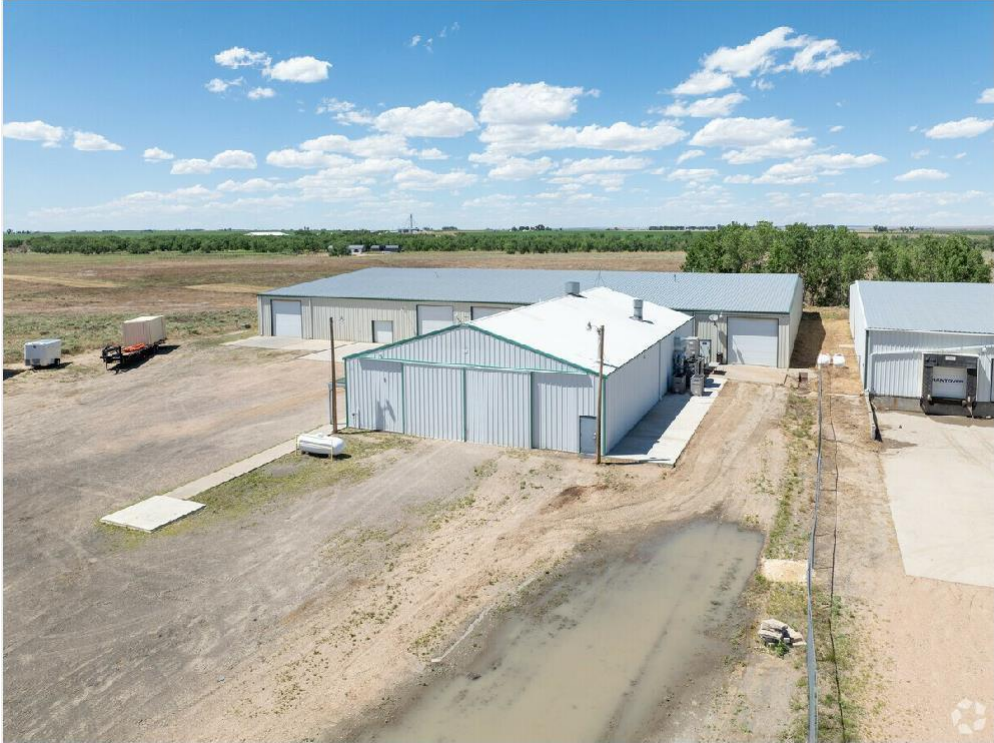
12555 ENERGY ROAD-AERIAL-EAST SIDE OF PROPERTY
