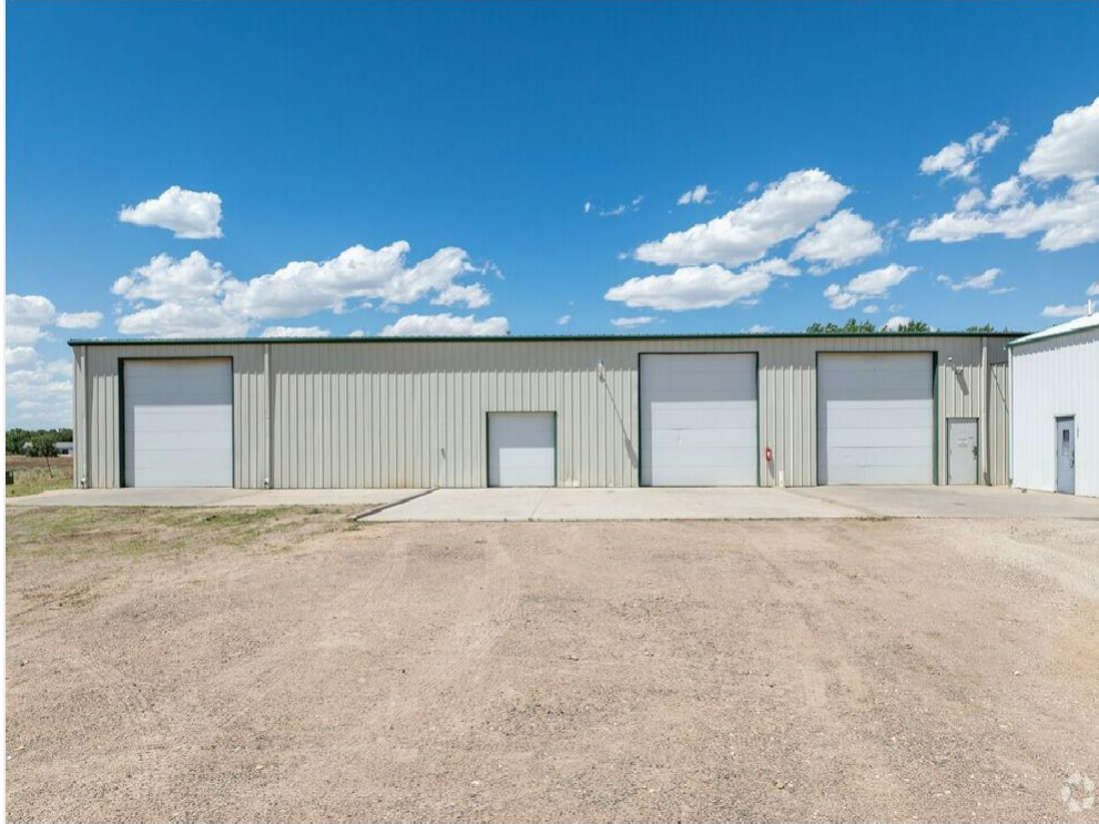
MAIN WAREHOUSE WITH CRANES/MACHINE SHOP
