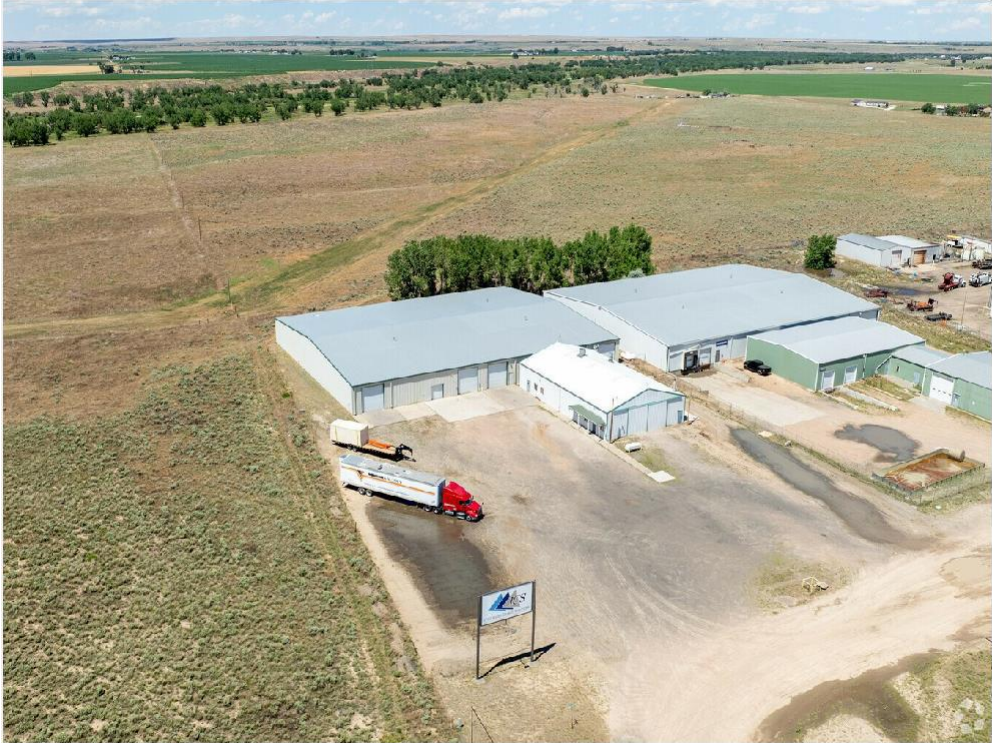
12555 ENERGY ROAD-AERIAL-WEST SIDE OF PROPERTY
