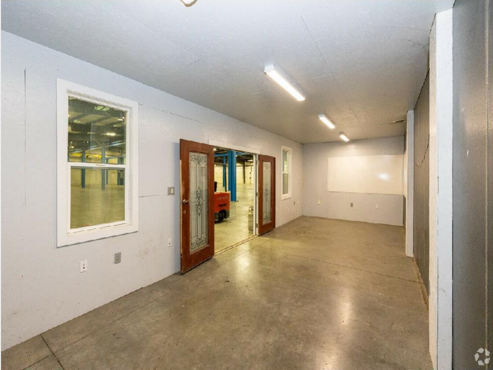
MAIN WAREHOUSE-BREAK ROOM/STORAGE ROOM/OFFICE SPACE (TEMP CONTROLLED)
