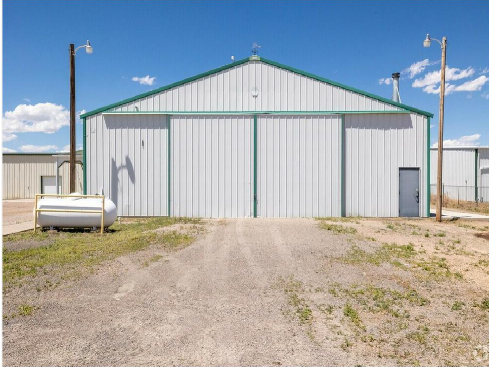
SECONDARY WAREHOUSE WITH PAINT BOOTH
