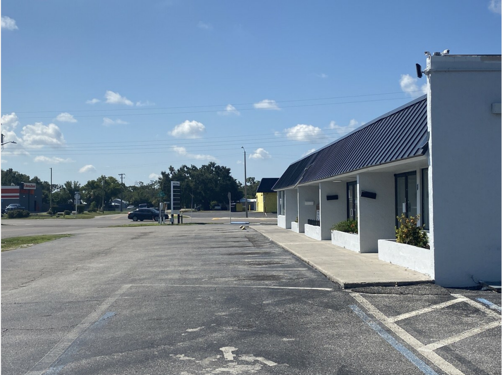
Exterior West Facing front parking
