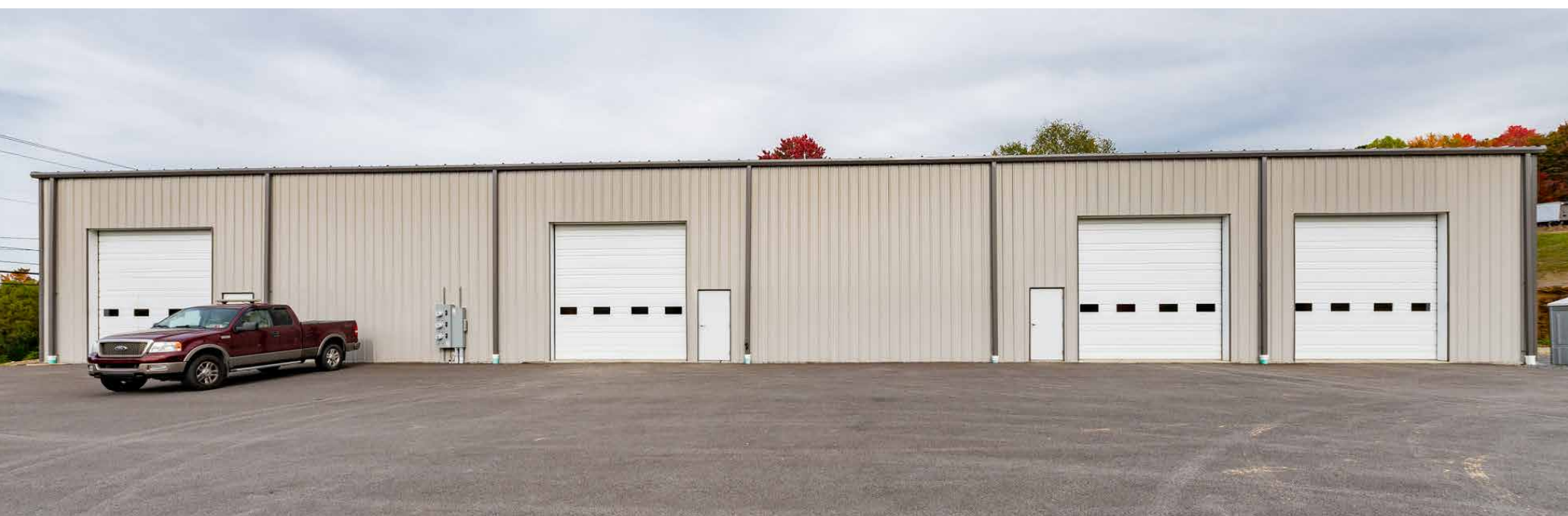
Front View of the Building.
