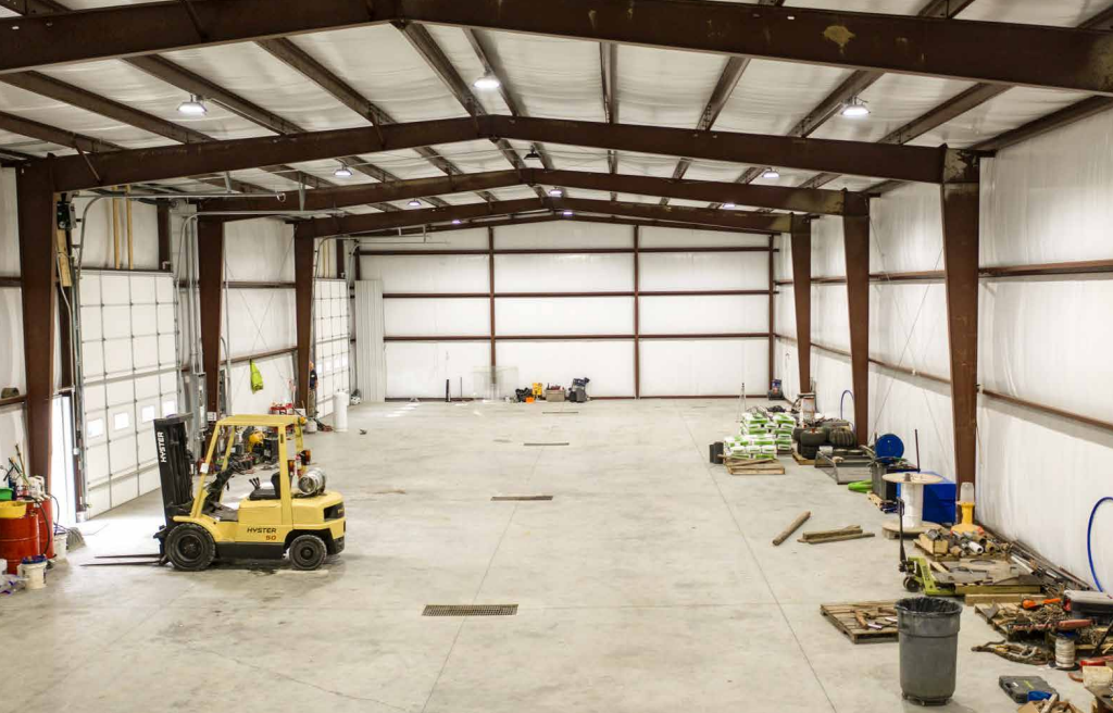
Interior Warehouse Area.
