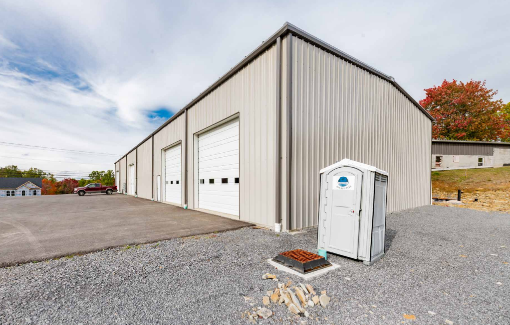
Front and Side View of the Building.
