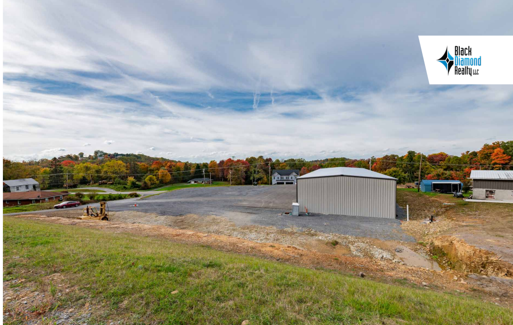
Elevated View of the Property Facing Fairchance Road.
