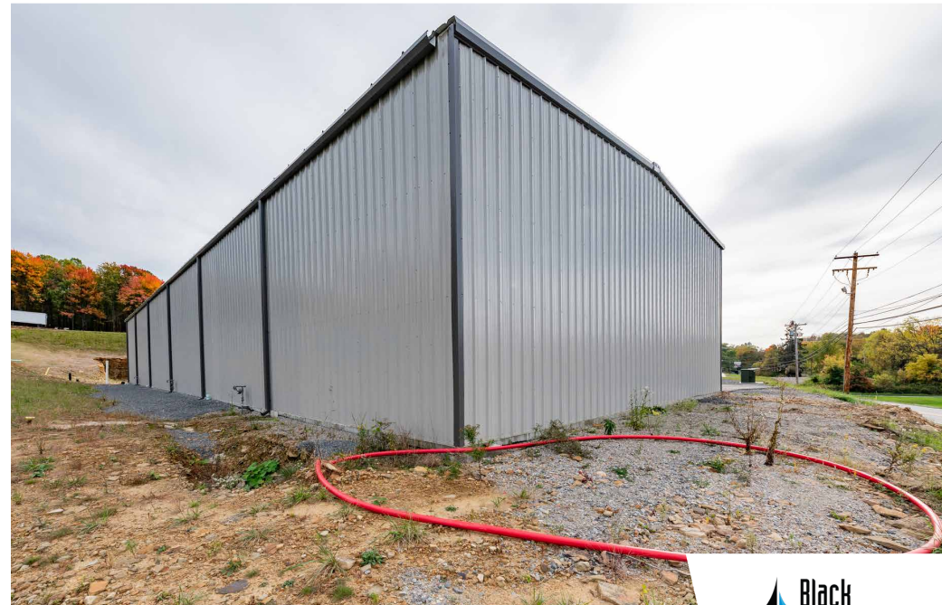
Back and Side of the Building.
