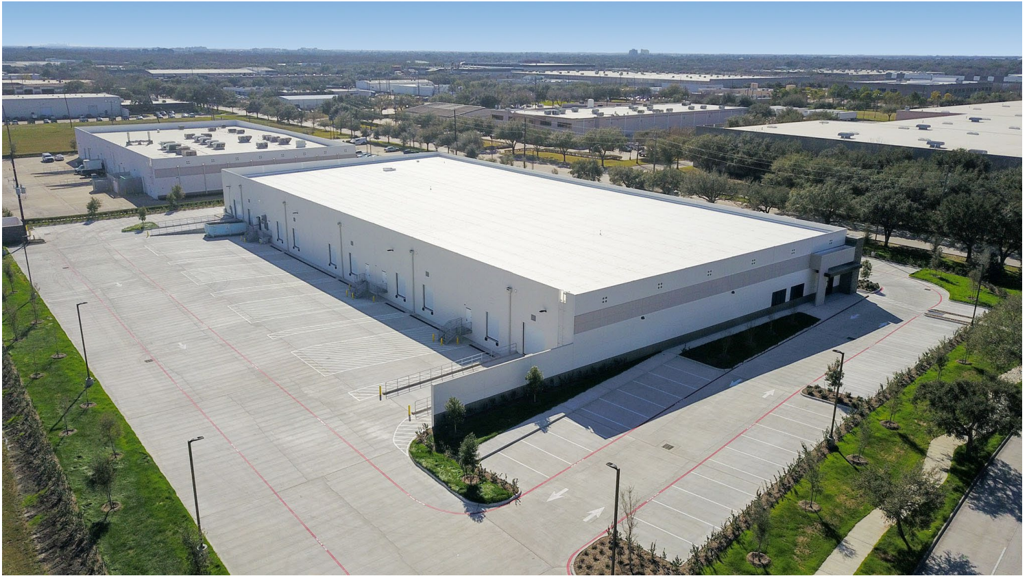
Aerial view of rear loading area
