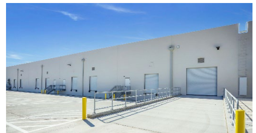
Rear Loading Area
