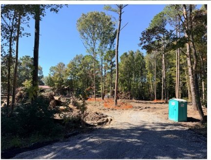
Land Clear and Underway
