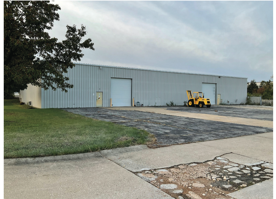
12,000 SF Manufacturing Building
