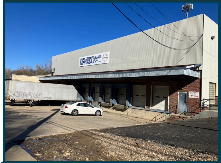
Lower Warehouse Loading
