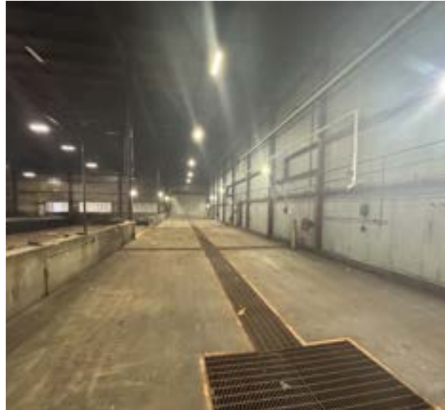
Drive through bay
