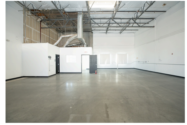
WAREHOUSE FACING OFFICE & RR
