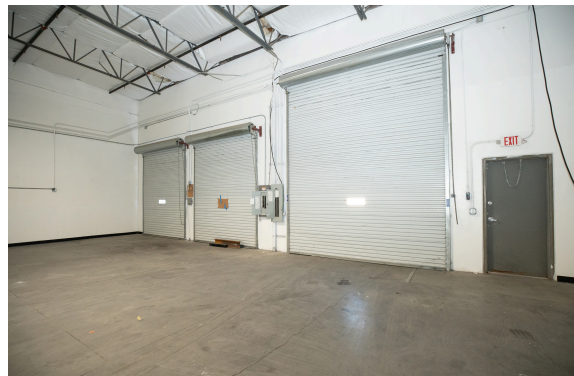
2 DOCK DOORS & 1 GRADE DOOR
