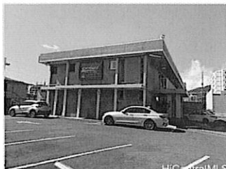
Front of building with 112 feet frontage on S. King St.
