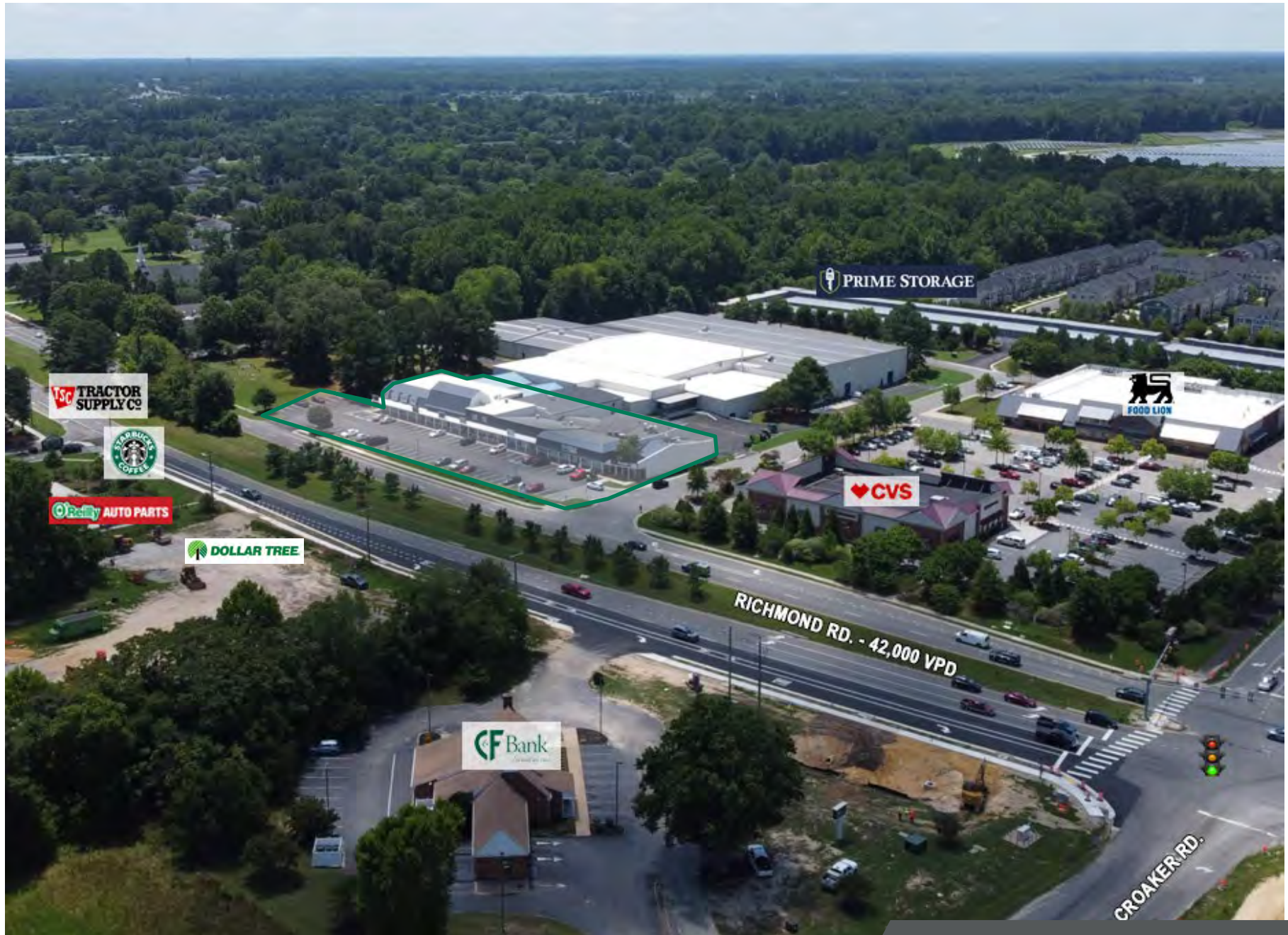
CANDLE FACTORY BUILDING 7521 RICHMOND RD., WILLIAMSBURG, VA
