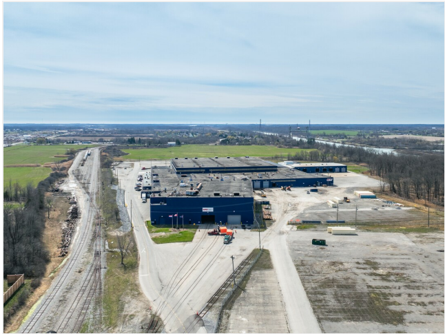
Thorold Hub - Hayes Road - Aerial
