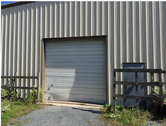
Building 1 At-Grade Door
