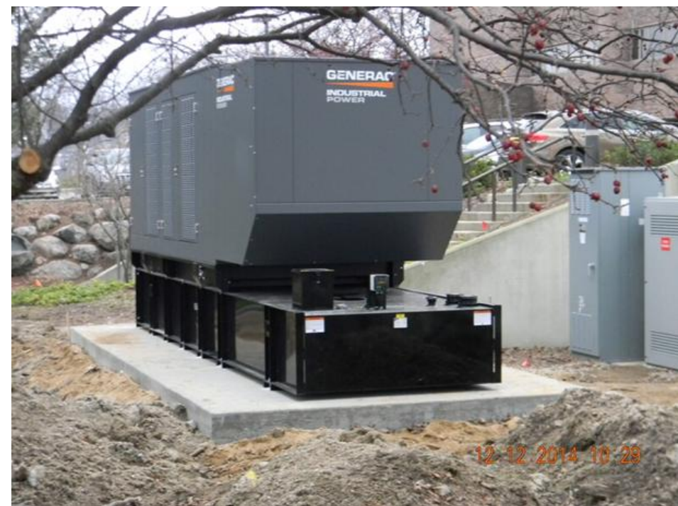
BUILDING WIDE BACK-UP GENERATOR
